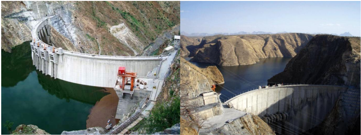
Figure 3.2: (a) Upstream and (b) Downstream view of Tekeze dam (Source, Inauguration report)
