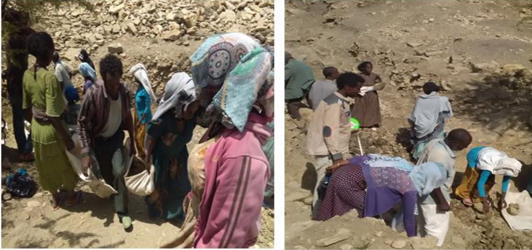
Fig 4.5 People of Tabia Aynalem Participating in Check dam construction
