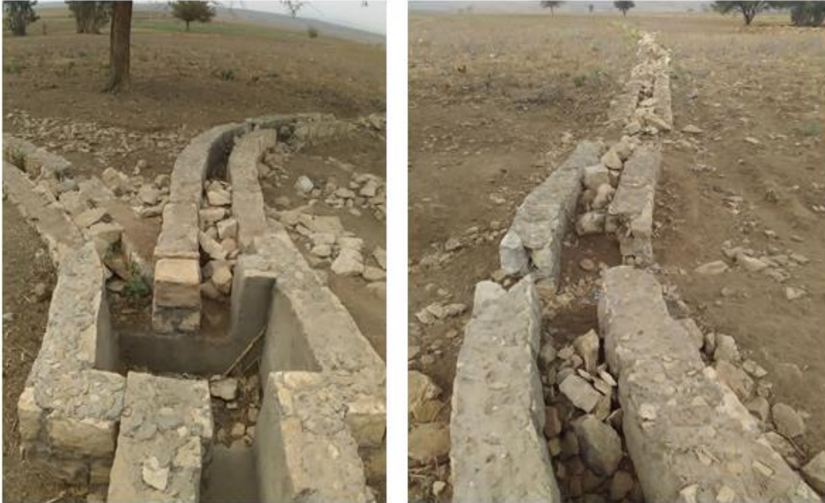
Fig 4.6 Destroyed but not maintained irrigation canal
