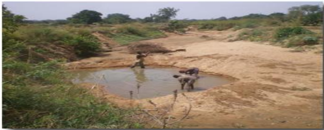
Figure 2.5: Alluvial dug out under construction
