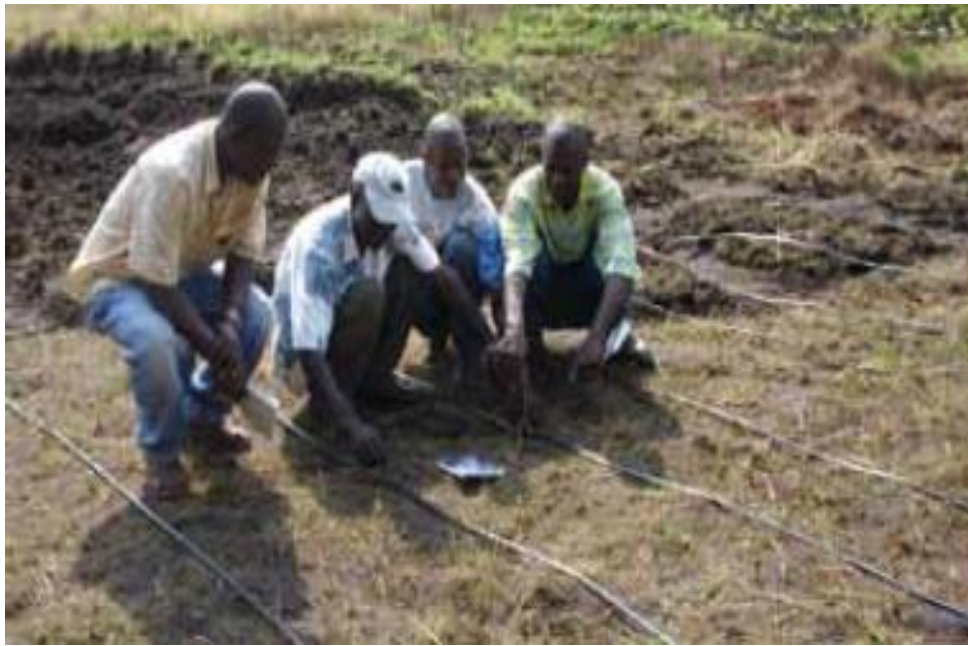
Figure 2. 9 Installation of drip irrigation lines
