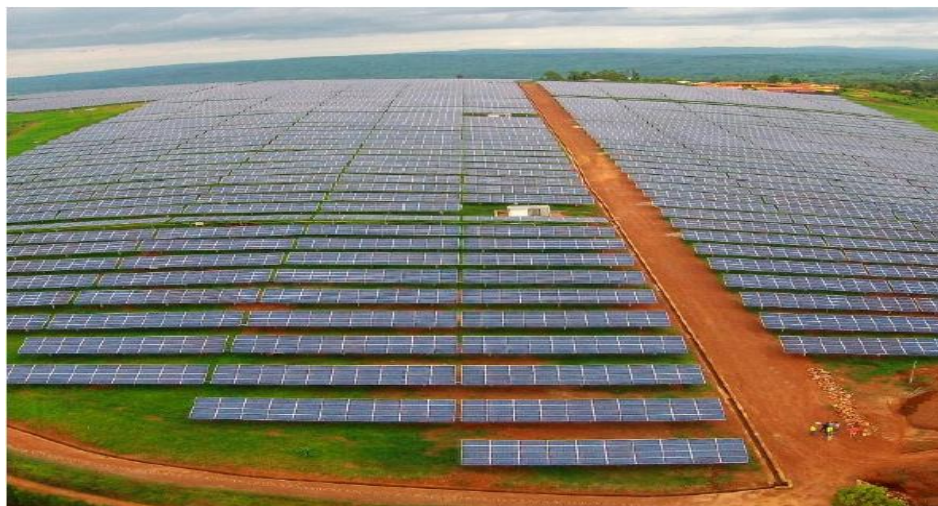
Figure 2. 6 : Utility-scale of 8.5MW PV power plant constructed in Agahozo-Shalom Youth Village in Rwanda.
