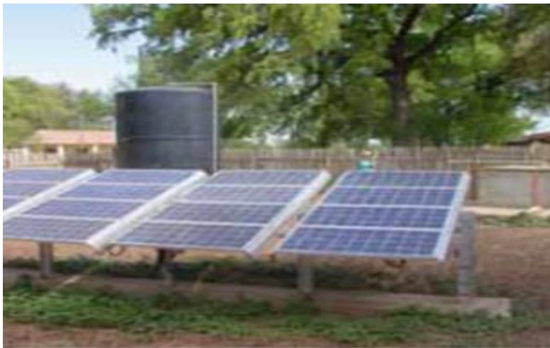
Figure 2. 2 Solar panels, pump and reservoir for drinking water and garden irrigation
