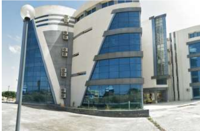
South west facade
