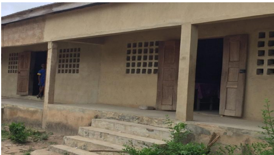
Figure 23: Donvagne primary school without electricity
