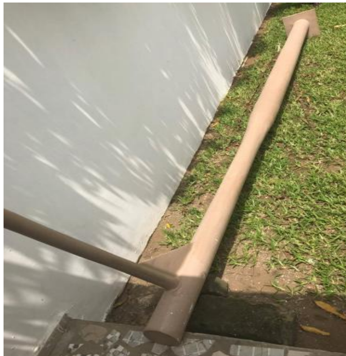
Figure 31: Light pole supports electric cables made out of 100 percent recycled plastic
