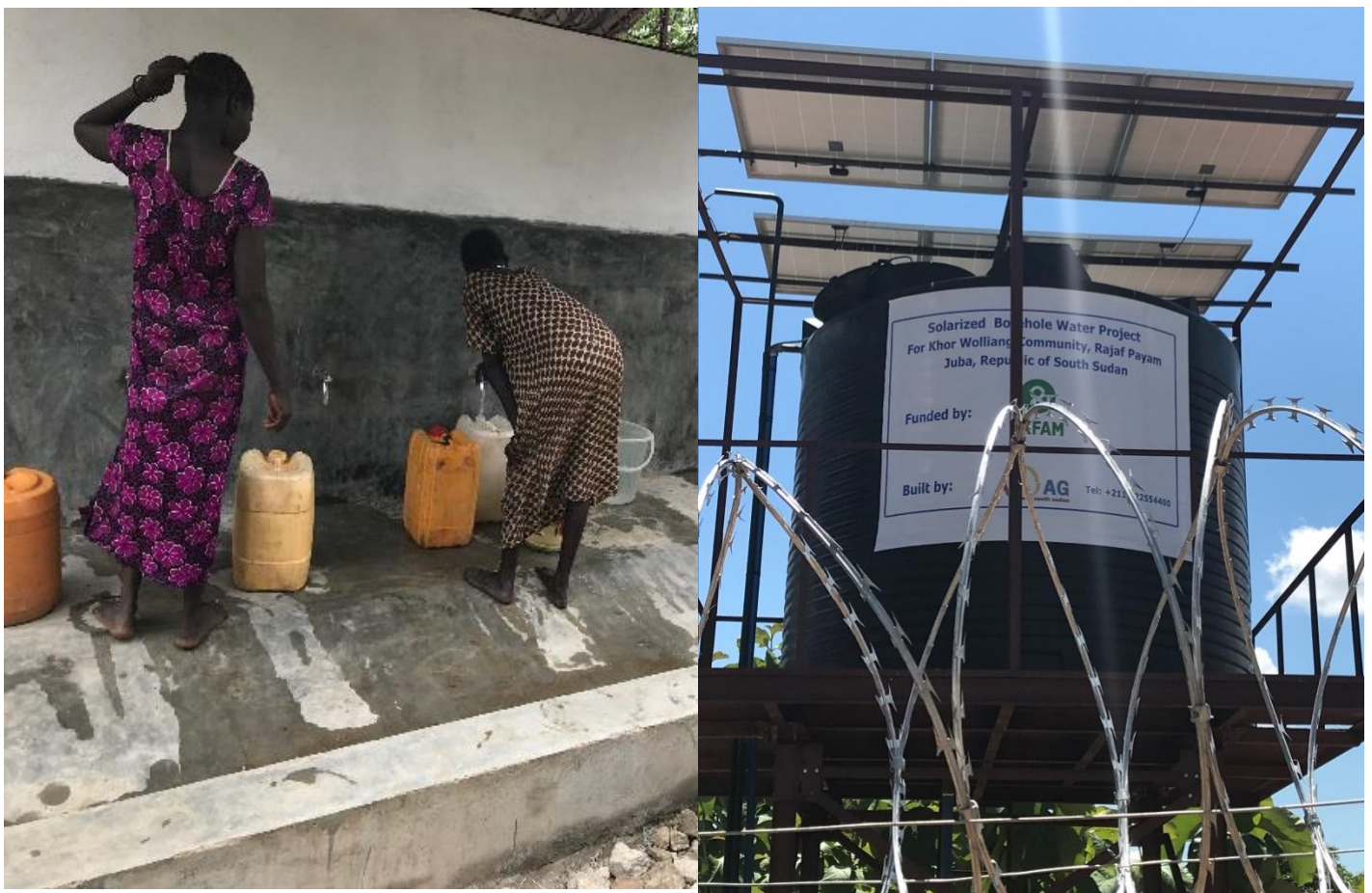
Fig 4.3; Showing a borehole built by Oxfam in Khor Williang community.
