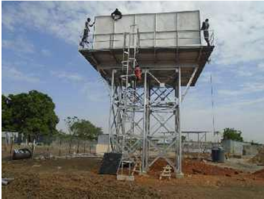
Figure 4.8 Elevated Water Tank
