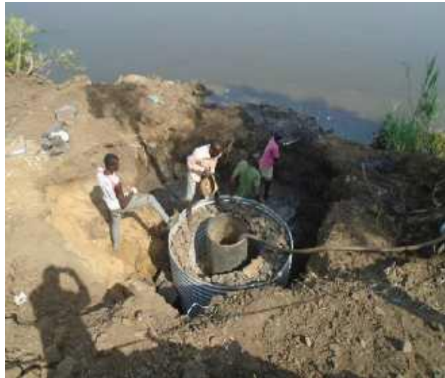
Figure 4.5. Showing the Filtration System
