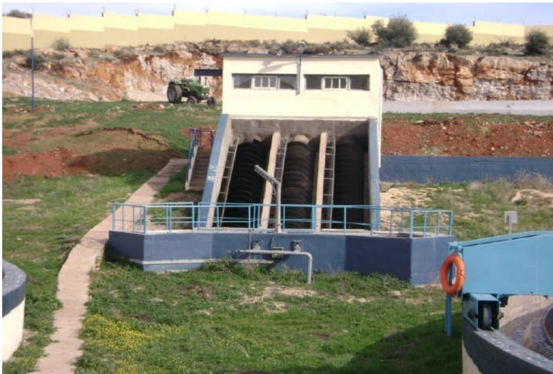
Figure 3.16 Sludge pumping
