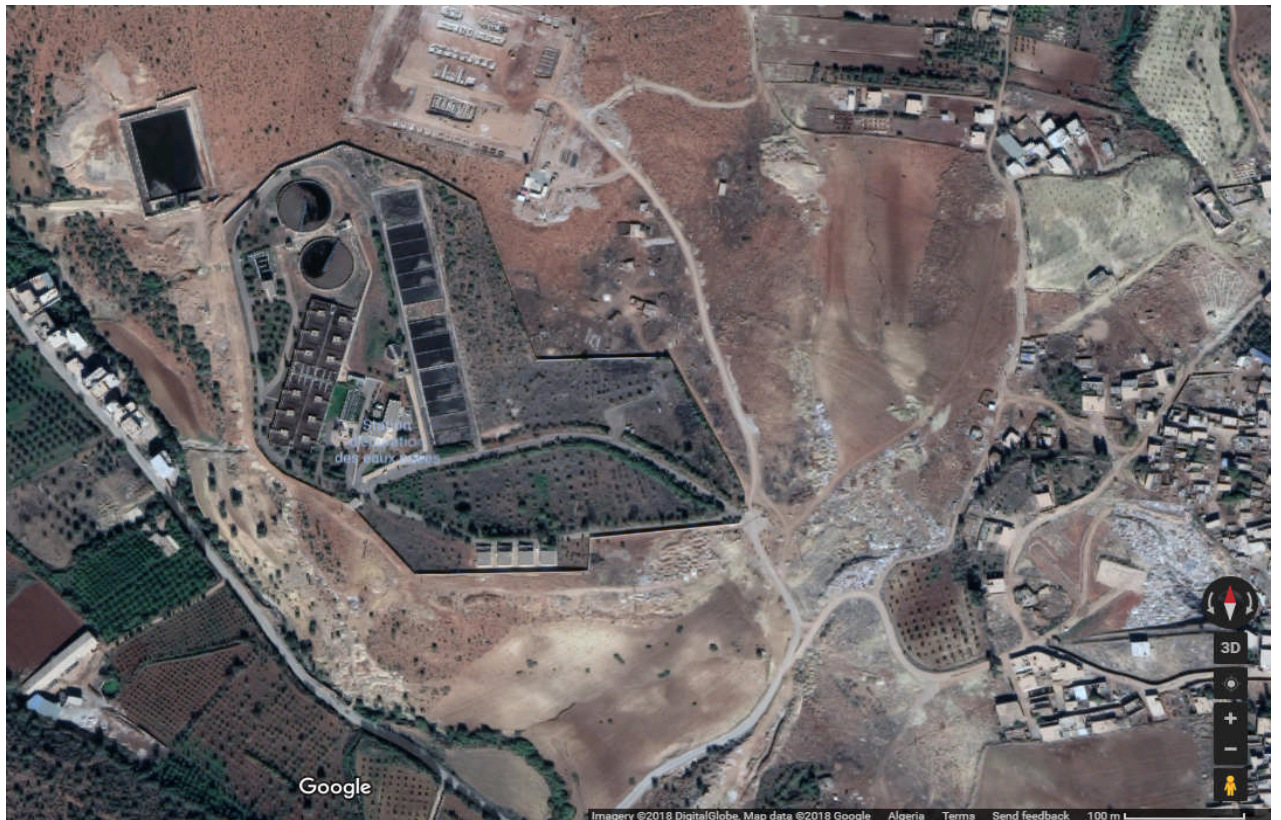
Figure 3.8 Ain El houtz wastewater treatment plant
