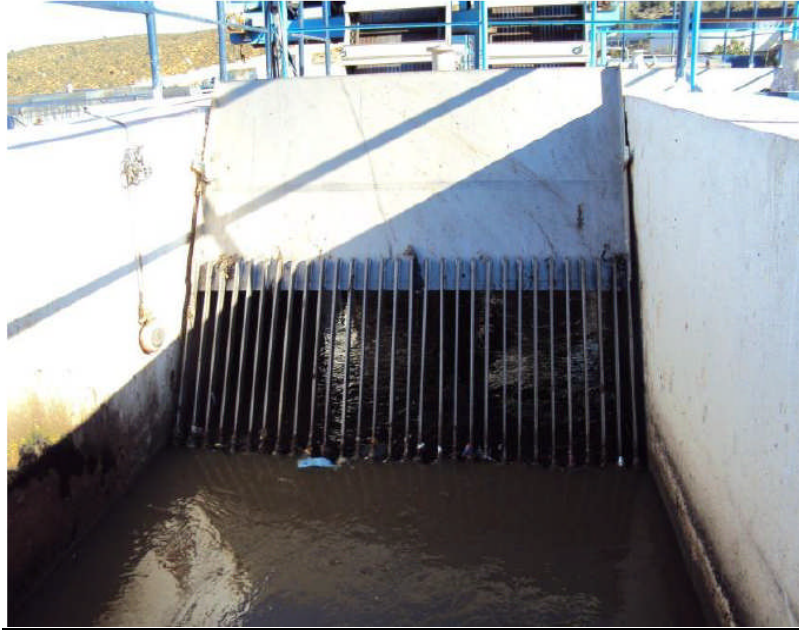
Figure 3.10 Traveling screen
