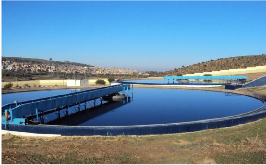
Figure 3.14 Secondary clarifier
