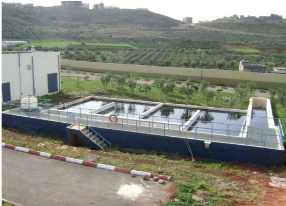
Figure 3.15 Chlorination tank
