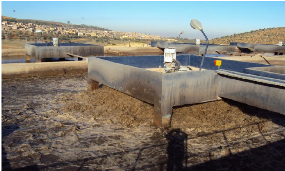
Figure 3.12 Aeration tank
