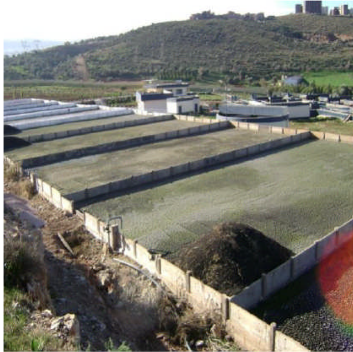
Figure 3.17 Sludge dryer
