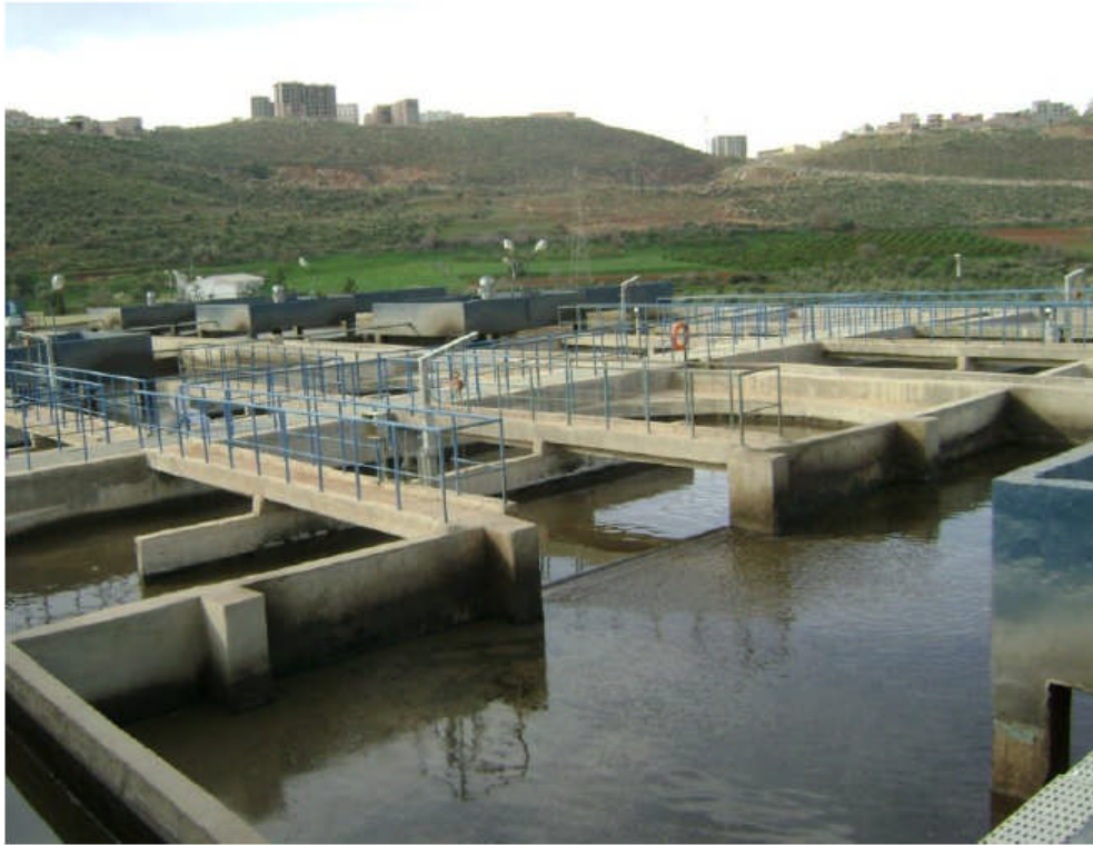
Figure 3.13 Nitrification denitrification tank
