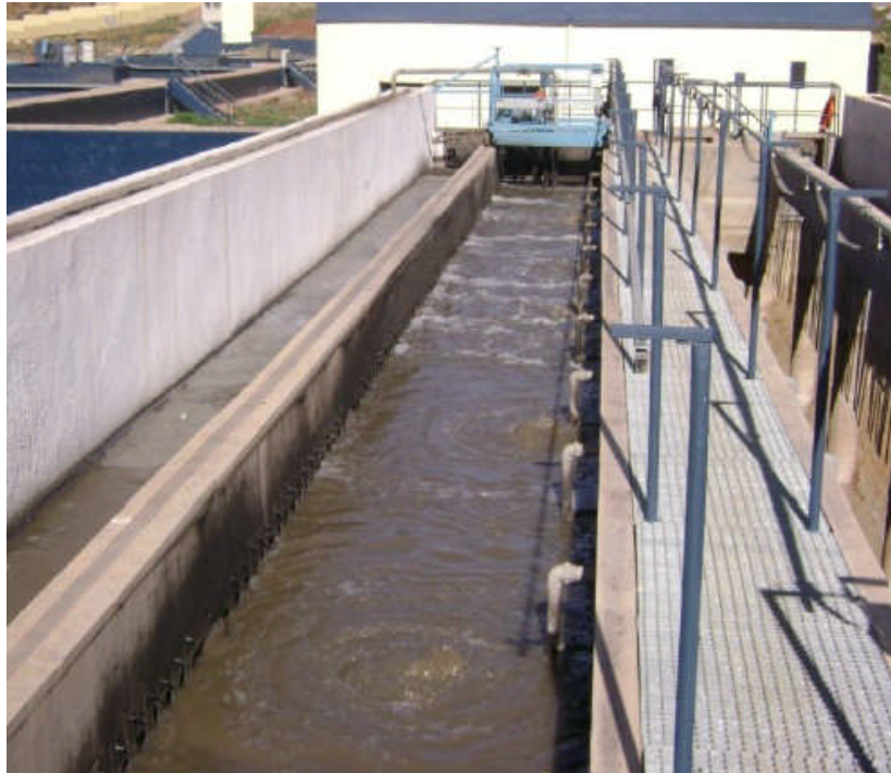
Figure 3.11 Sand trap
