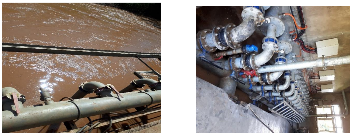
Figure 4.12: Water pumping from Umuvumba river/Kagitumba irrigation site
