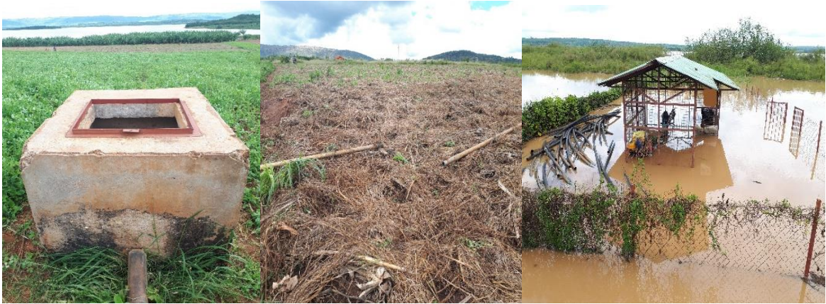
Figure 4.21: Irrigation infrastructures damaged (Gashora and Nasho/Mpanga irrigation sites)
