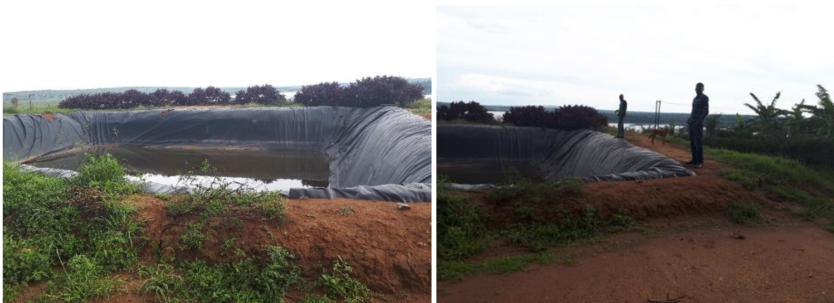
Figure 4.11: Dam sheet/Gashora irrigation site
