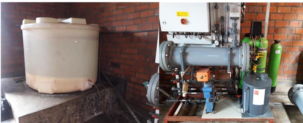
**Preparation of Chlorine disinfectant by electrolysis of sodium chloride**
