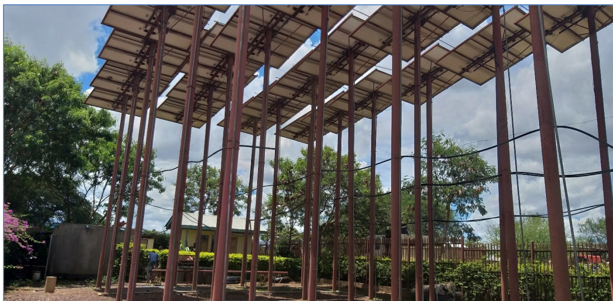
Figure 4. 3 A 27.6 kW array installed at Kiruha-Kahe
