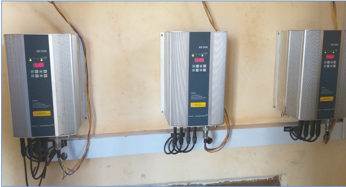
Figure 4. 4 Three installed inverters at the SWP station
