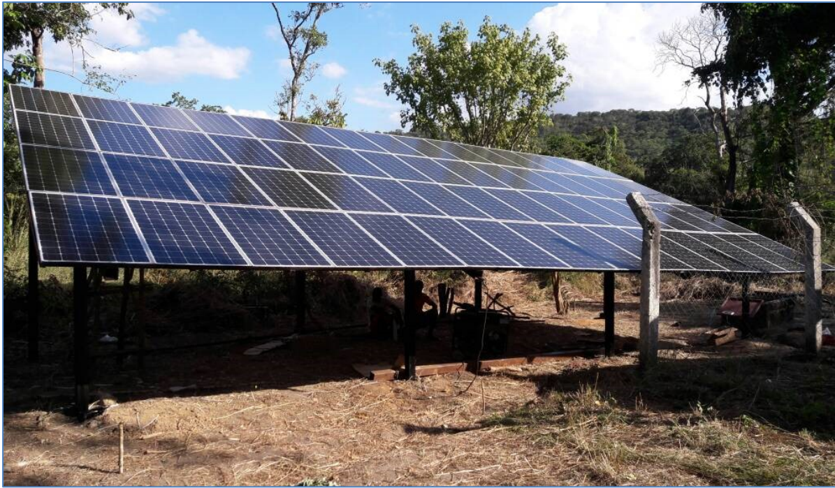
Figure 4. 23 Connected solar array in Nanyamba district
