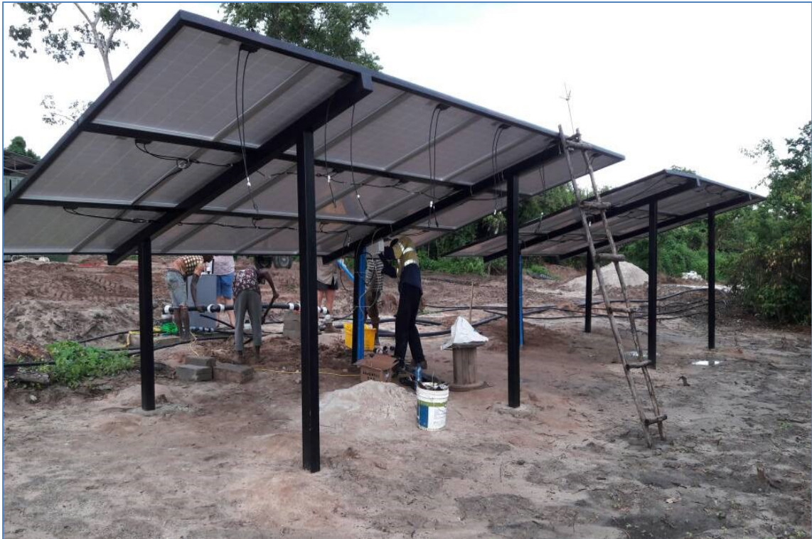
Figure 4. 22 Fixed solar panels on top of support structures
