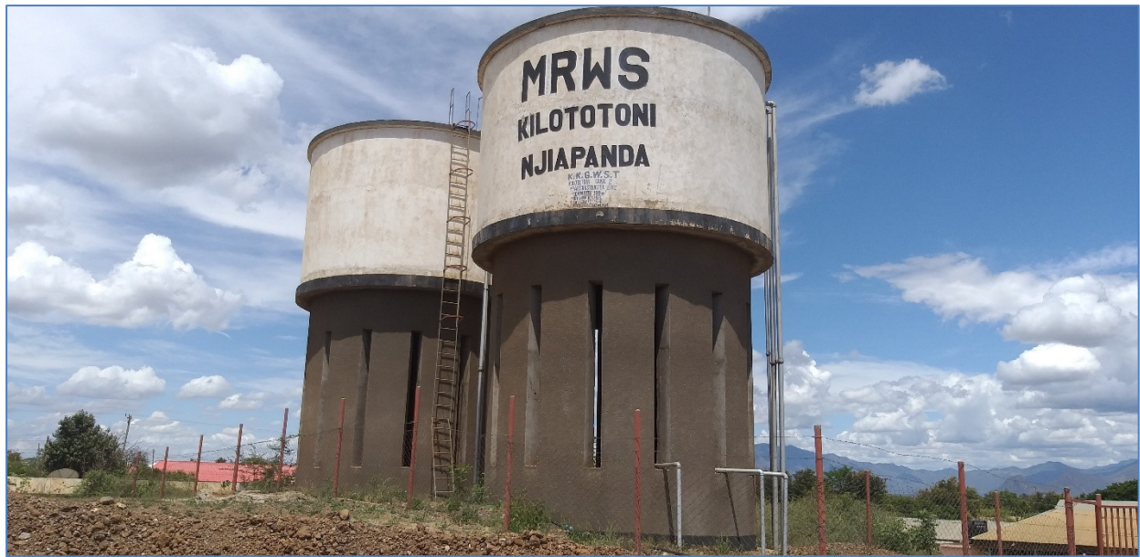
Figure 4. 6 Storage water tanks
