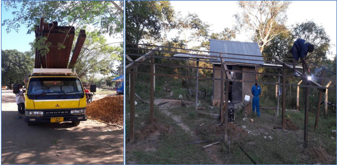
Figure 4. 21 Transporting and Installing Solar structure supports
