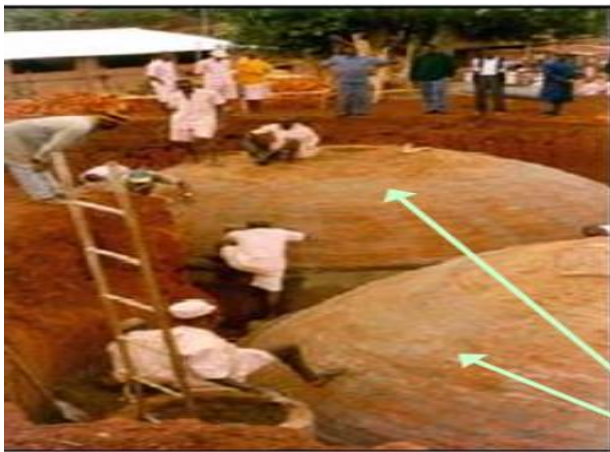
Figure 5. Biogas digester at CYANGUGU prison (Butare and Karamo,2002)
