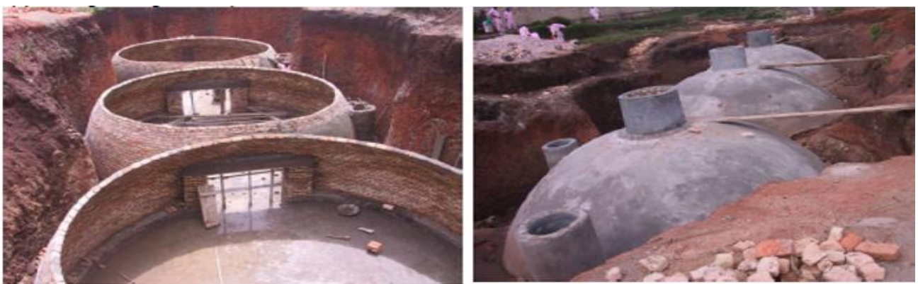
Figure 4. Digesters under construction at NSTINDA prison (source: OXFAM,2011)
