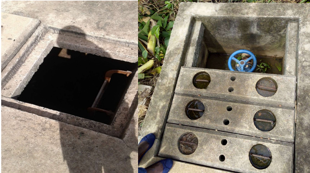
Figure 4-1: Status of the manholes
