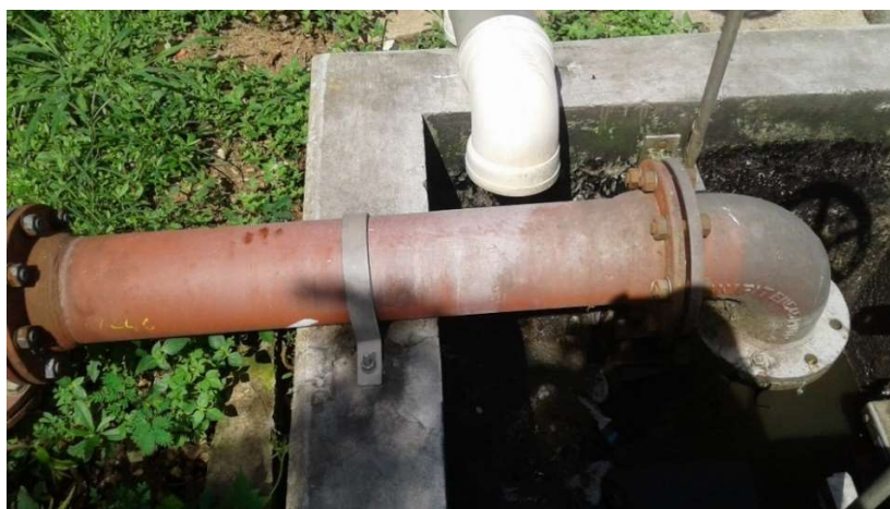
Figure 4-2: KNUST sewerage network conducts
