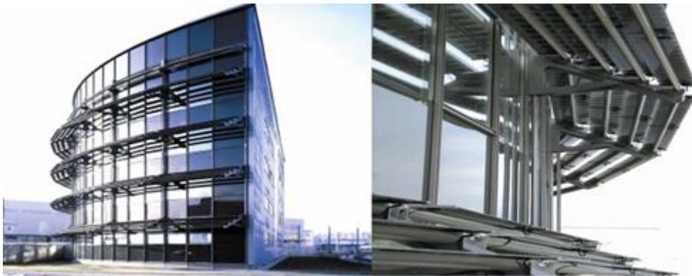
Figure 25:SBL Offices Linz, Austria, Helmut Schimek, shading louvers with integrated photovoltaics and suntracking system, © Colt
