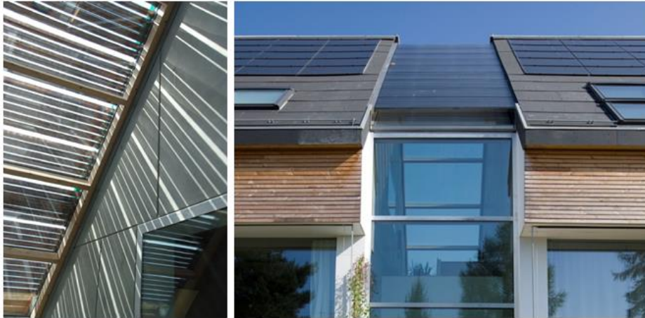
Figure 40: Evacuated tubes collectors used as glazed roof sunshading (left: inside view, right: outside view) (Dubendorf Residential building, Beat Kaempfen 2008).
