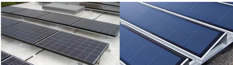
Figure 16:crystalline modules for flat roof. Left: standard module on rack mounting system, © Prosolar
