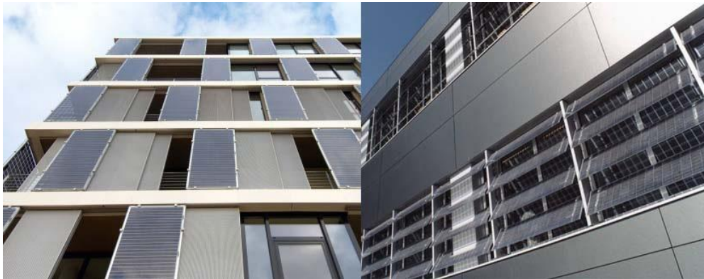
Figure 24:solar shading solution: Left: Colt Ellisse PV sliding shades at Company HQ, Bitterfeld-Wolfen, Germany, © Colt, Right: Keuringsdienst, Eindhoven, The Netherlands, Yanovshchinsky Architekten: using Colt Shadovoltaic as shading device, © Colt.
