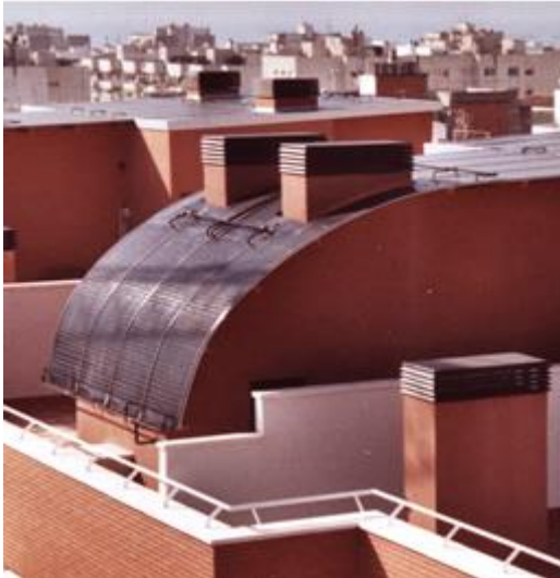
Figure 37: Roof integration of unglazed flat plate collectors used as roof covering (Energie Solaire SA).
