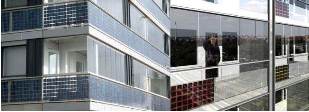
Figure 26; spandrels and parapet solutions. Left: Housing Estate, Ekovikki, Finland, Oy Reijo Jallinoja: semi-transparent PV modules with two-paned glazing in parapet areas, Resource: PV NORD. Right: Kollektivhuset, Copenhagen, Denmark, Domus Arkitekter: PV cells
