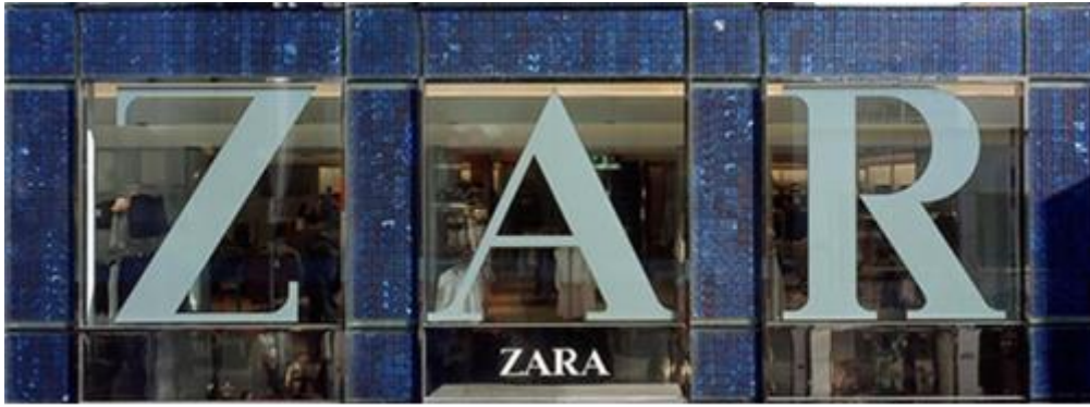
Figure 21:warm façade solution. Zara Fashion Store, Cologne, Germany, Architekturbüro Angela und Georg Feinhals: opaque monocrystalline cells combined with transparent glazing in post-beam curtain wall structure, © Solon.
