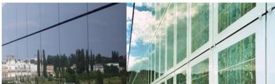
Figure 20: A Facade cladding solutions. Left: Solteature Solartechnik GmbH, Berlin, Germany, © Solteaturel. Right: Paul-Horn Arena, Tübingen, Germany, Alman-Sattler-Wappner, © Sunways.
