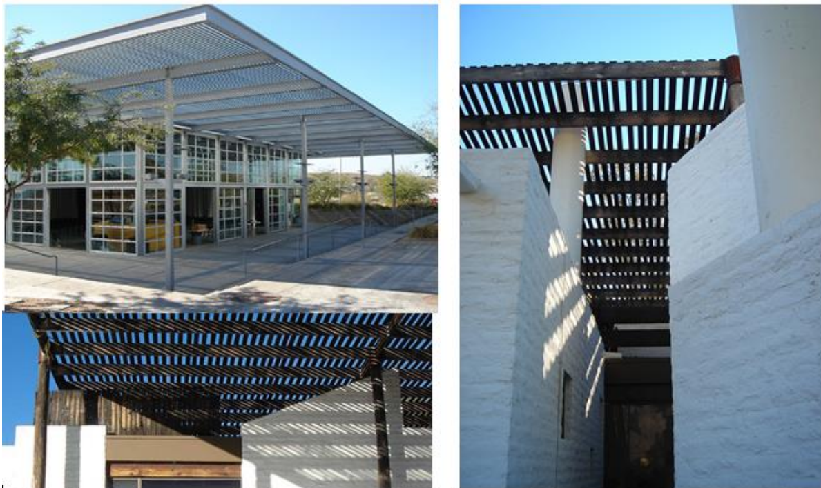
Figure 41: Examples of double roofs conceived to reduce building heat (a: double tin roof in Arizona architect n.a; b and c: double roof on a private house in Arizona (Architect Judit Chafee, credits Marja Lundgren).
