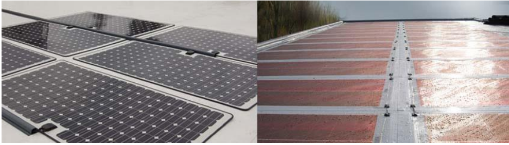
Figure 17: integration of thin film laminates on flexible substrate in flat roof.
