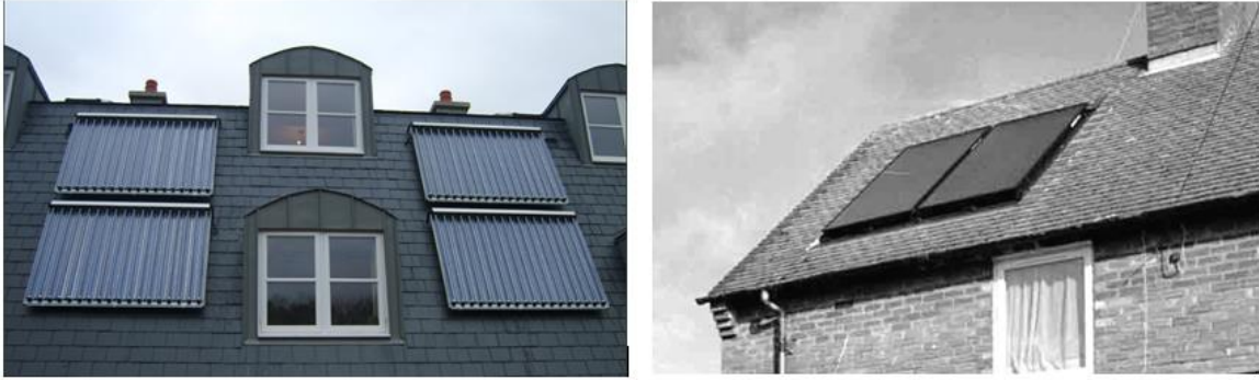
Figure 33: Integration of collectors as added elements on the roof.
