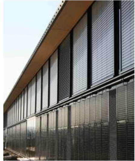
Figure 36: Façade integration of unglazed flat plate collectors used as façade cladding.
