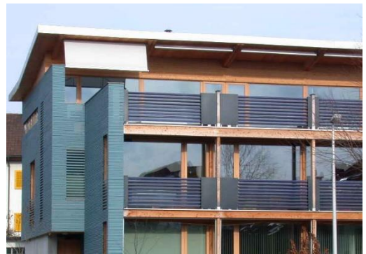
Figure 38: Evacuated tubes collectors used as balcony eaves
