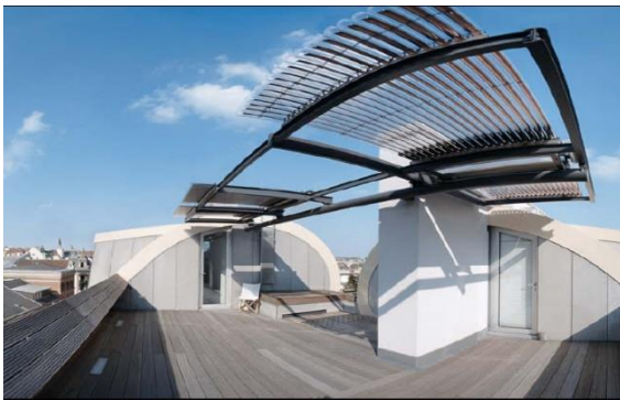
Figure 39: Evacuated tubes collectors used as deck sun shading (RaU Architekten)
