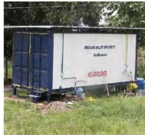
Figure 2.1b. Dry digestion pilot plant at KNUST, Kumasi, Ghana ([24])
