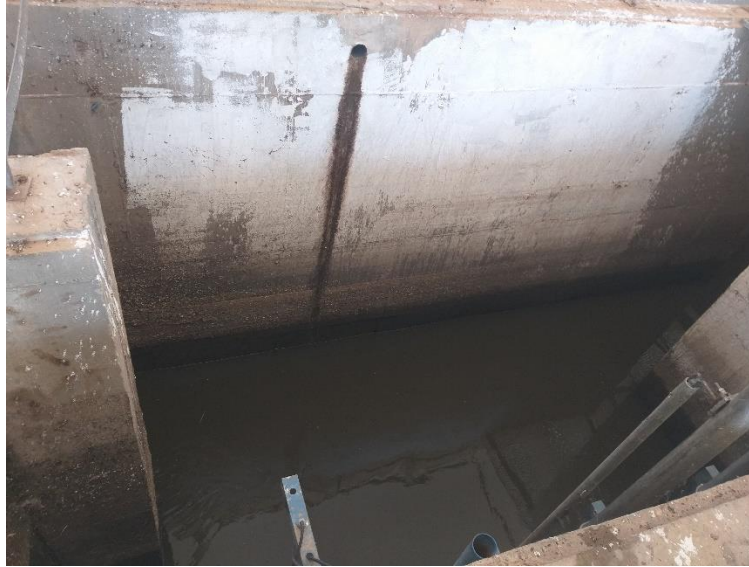
Figure IV.6: The sand trap (Source: WWTP of Ain Temouchent, 2020)
