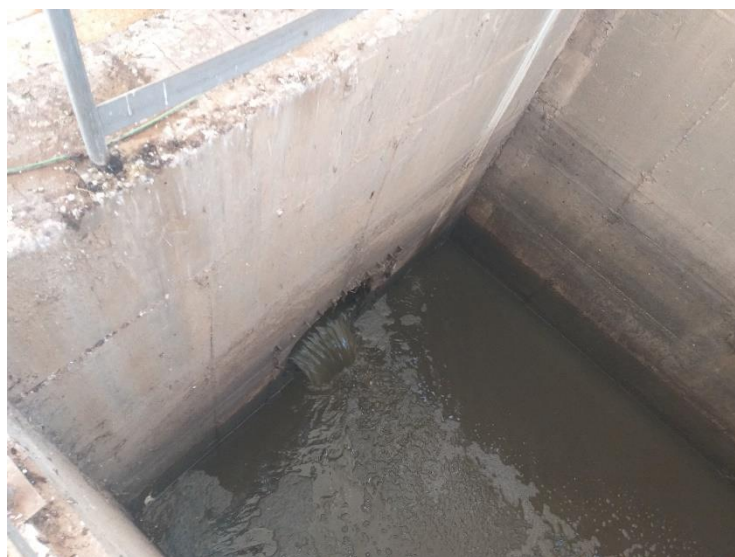
Figure IV.3: wastewater inlet in the WWTP (Source: WWTP of Ain Temouchent, 2020)
