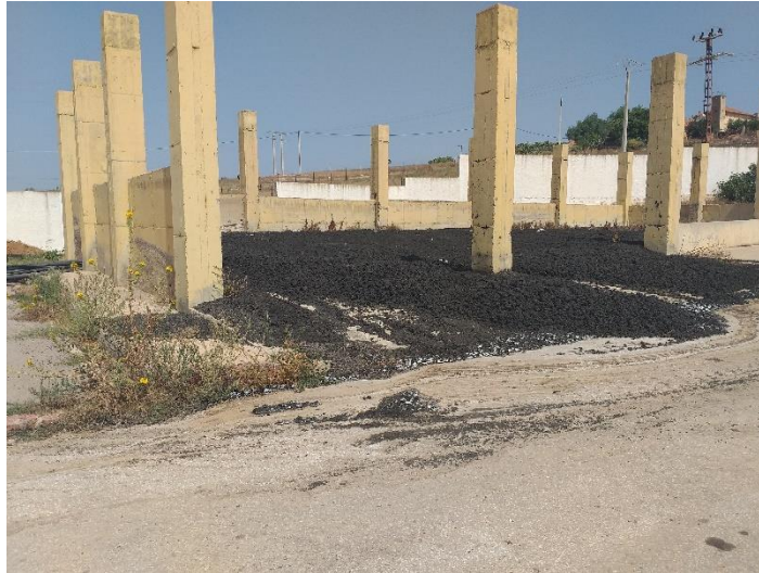
Figure IV.18: Drying beds (Source: WWTP of Ain Temouchent, 2020)
