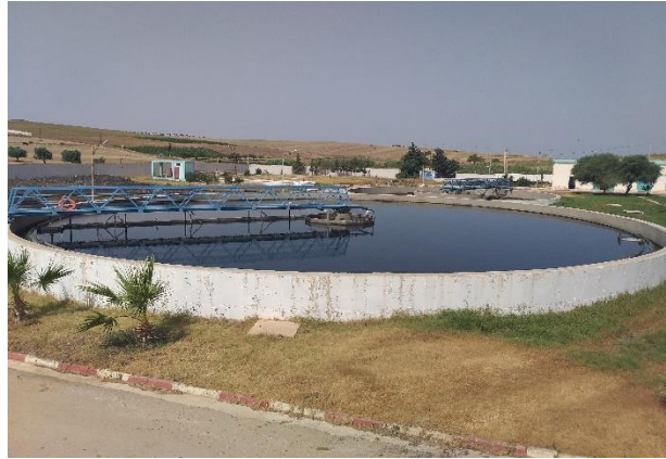
Figure IV.13: A secondary clarifier (Source: WWTP of Ain Temouchent, 2020)
