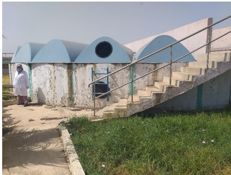
Figure IV.16: Sludge thickener (Source: WWTP of Ain Temouchent, 2020)
