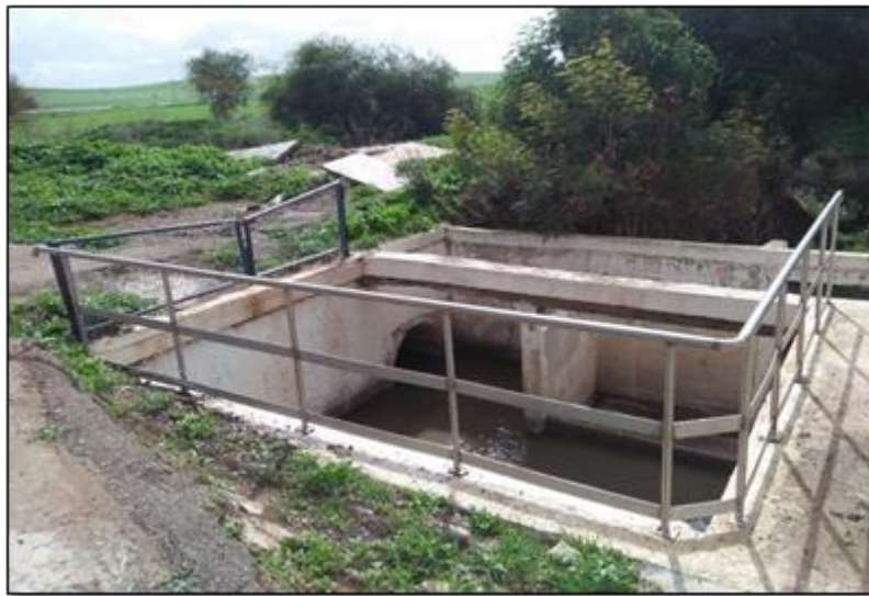
Figure IV.2: The Storm weir (Source: WWTP of Ain Temouchent, 2020)
