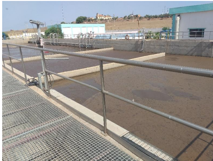
Figure III.12: Aeration basins for nitrification (Source: WWTP of Ain Temouchent, 2020)
