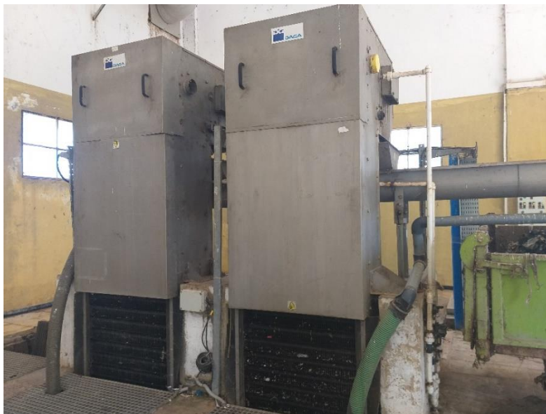
Figure IV.7: Fine Mechanical bar screens (Source: WWTP of Ain Temouchent, 2020)
