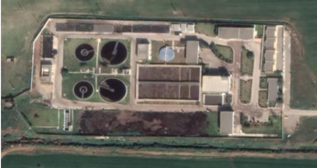
Figure 2: Geographical location of the WWTP
