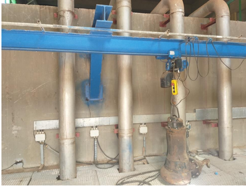
Figure IV.9: The lifting station (Source: WWTP of Ain Temouchent, 2020)
