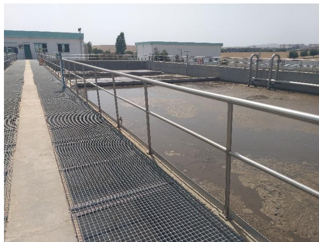
Figure IV.11: Aeration basins for denitrification (Source: WWTP of Ain Temouchent, 2018)
