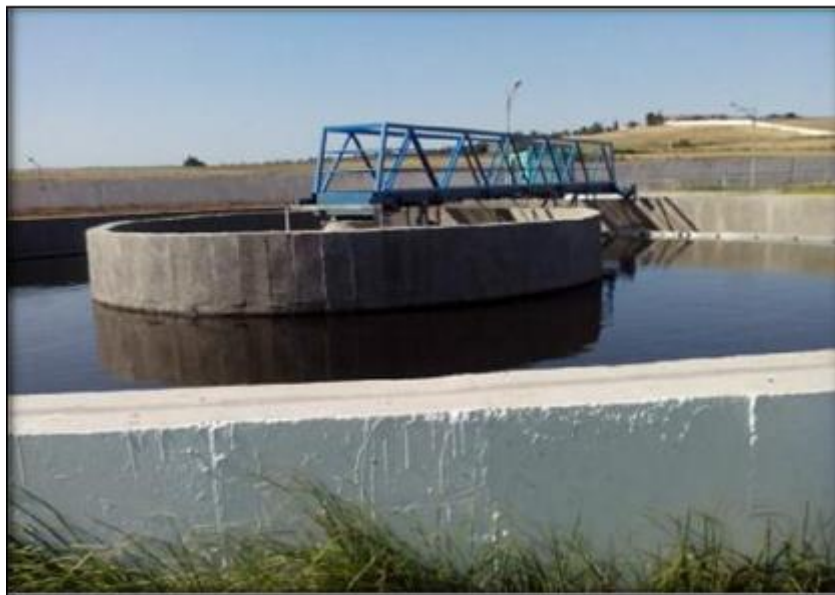
Figure IV.15: A clarifloculator (Source: WWTP of Ain Temouchent, 2020)
