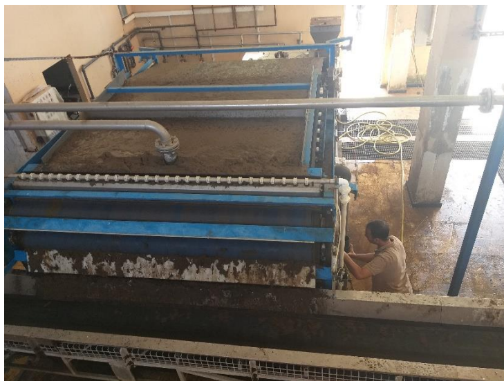
Figure III.19: Sludge dewatering belt press (Source: WWTP of Ain Temouchent, 2020)
