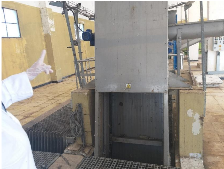
Figure IV.5: The coarse mechanical bar screen (Source: WWTP of Ain Temouchent, 2020)
