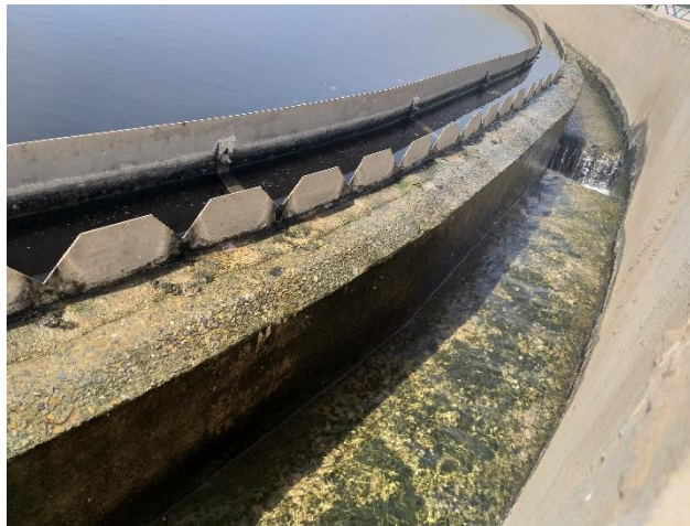
Figure IV.13: Treated wastewater flowing from the clarifiers (Source: WWTP of Ain Temouchent, 2020)
