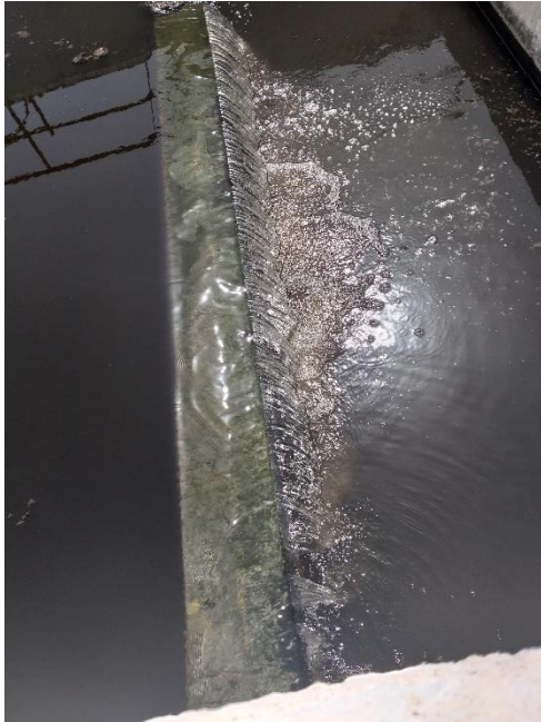
Figure IV.15: The disinfection basin (Source: WWTP of Ain Temouchent, 2018)
