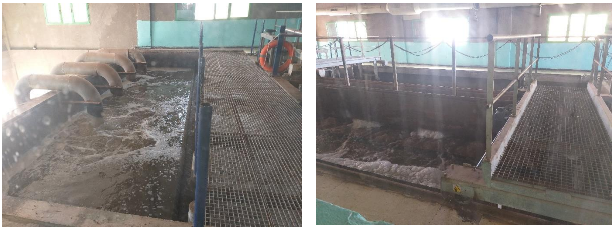
Figure IV.10: Sands, grease and oil removal units (Source: WWTP of Ain Temouchent, 2020)
