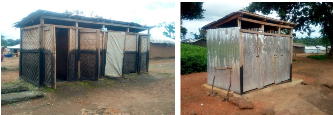
Photo 2: Different type of sanitary installation
