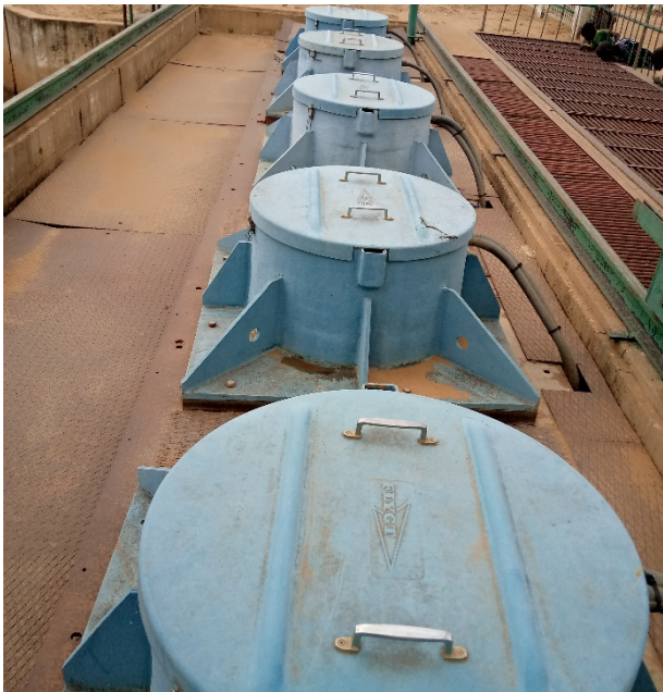
5 pumps of 600 m 3 /s Capacity at station 1
