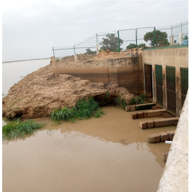
Pumping out point from the Logone River
