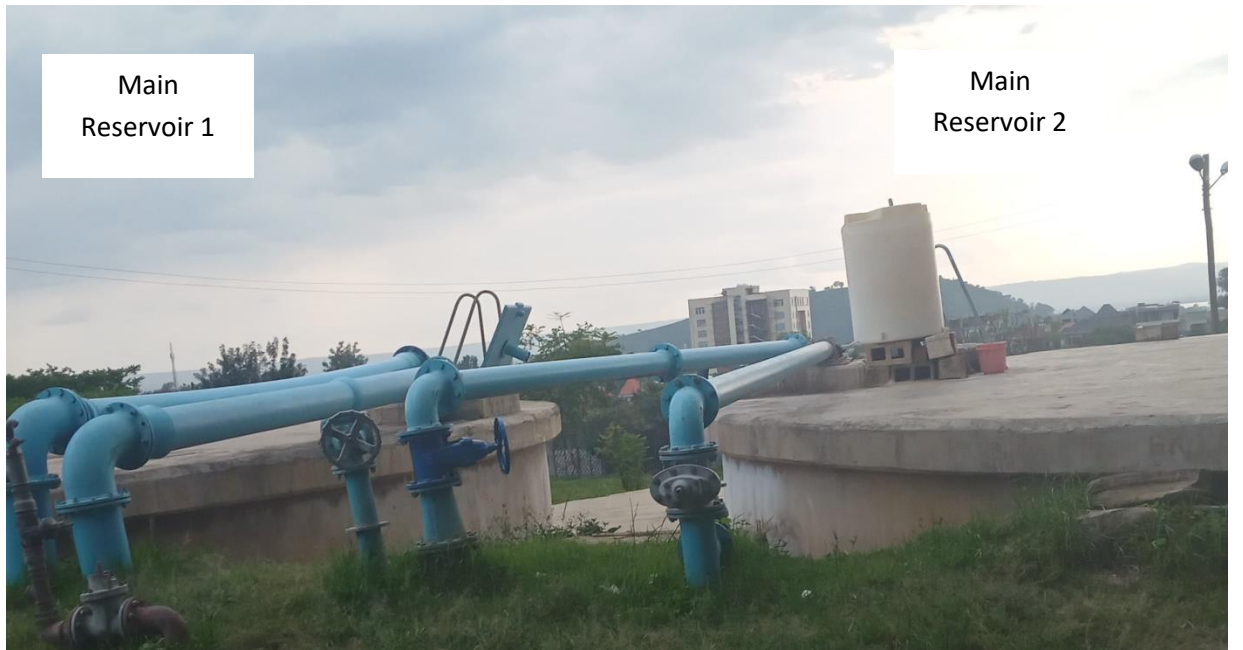
Figure: Hawassa water supply Reservoirs
