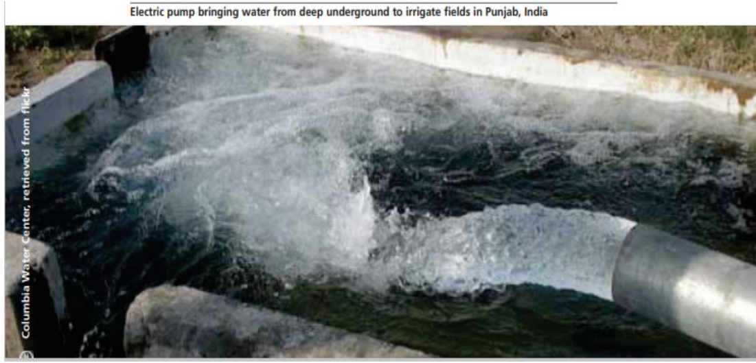
Figure 2.4: Electric pump bringing water from deep underground in India
