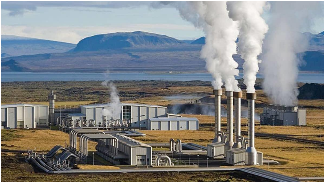
Figure 2.11. Lake Ngozi Geothermal Plant (Source: Construction review online)
