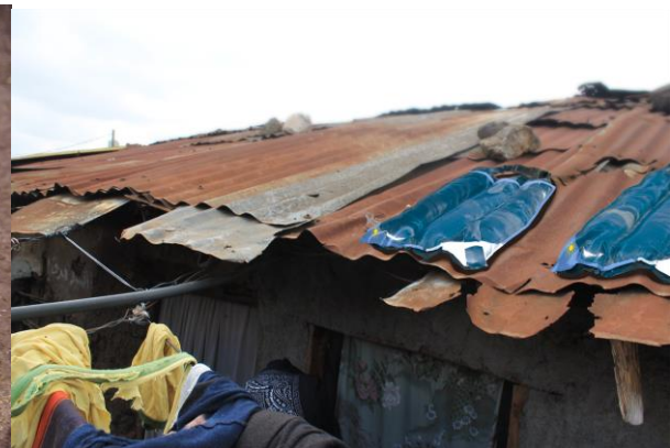
SolarSacks on the roof Kibera slum in Kenya
