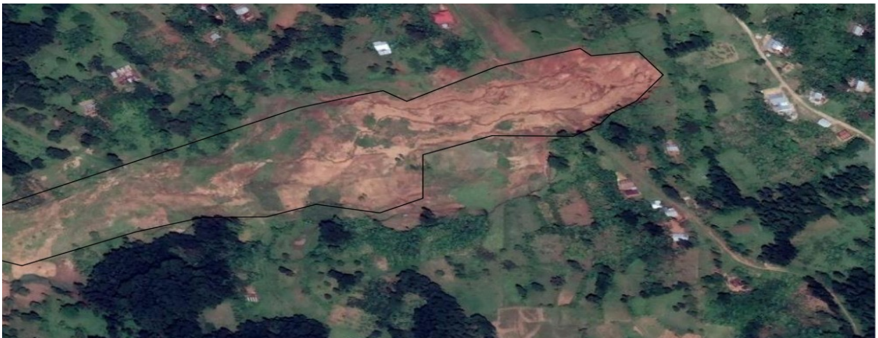
Figure 4-5: Google Satellite capture of one of the landslide Scars on 20 th September, 2021
