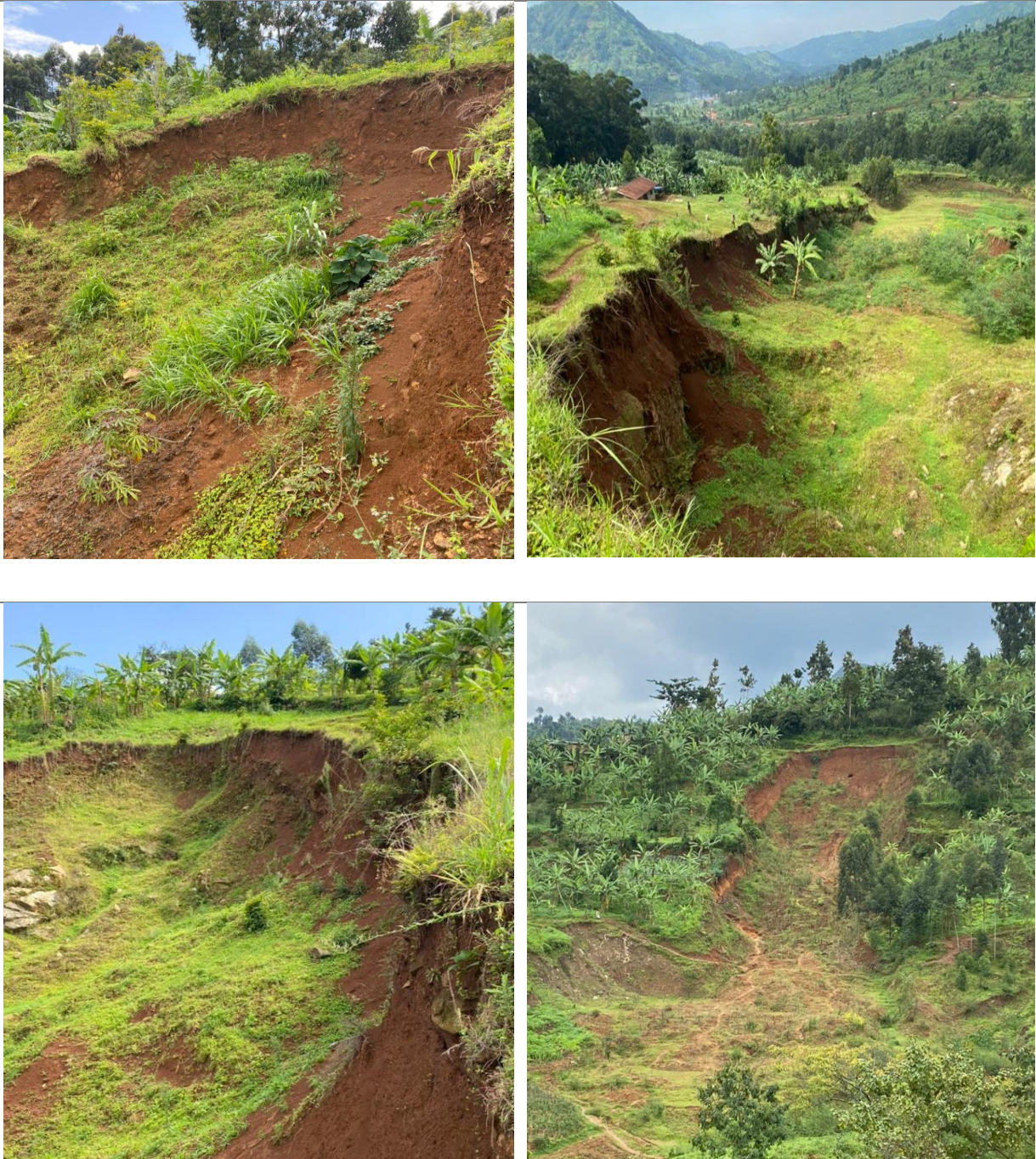
Figure 4-12: Landslide hotspots identified during the field visit
