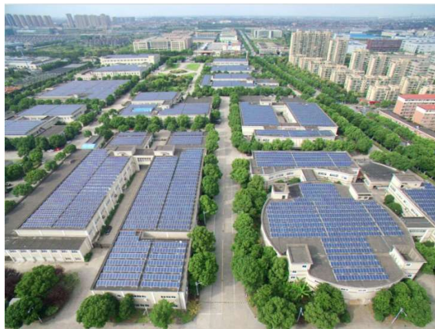
Figure 7.3: Rooftop solar PV installations.
