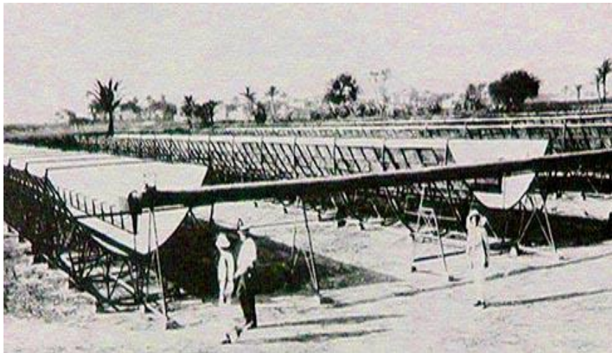
Figure 2.6: Parabolic trough driven pumping system
