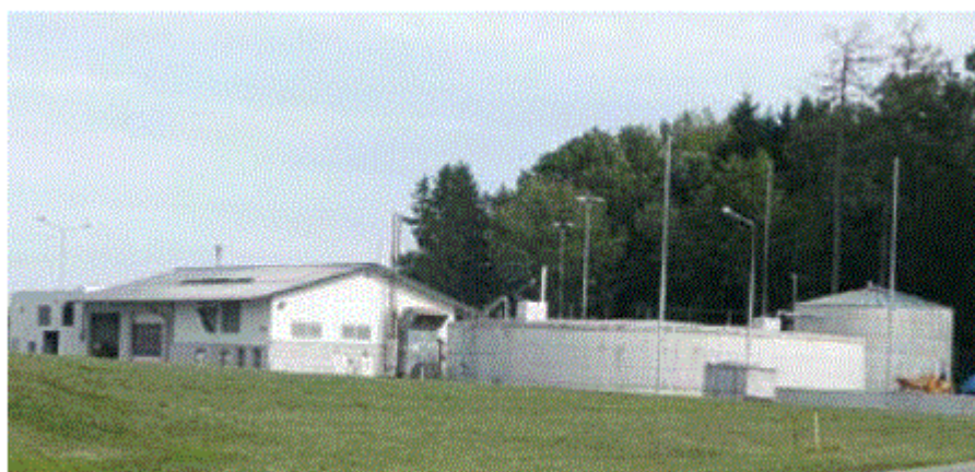
Figure 2.18. Biogas plant at St. Martin
