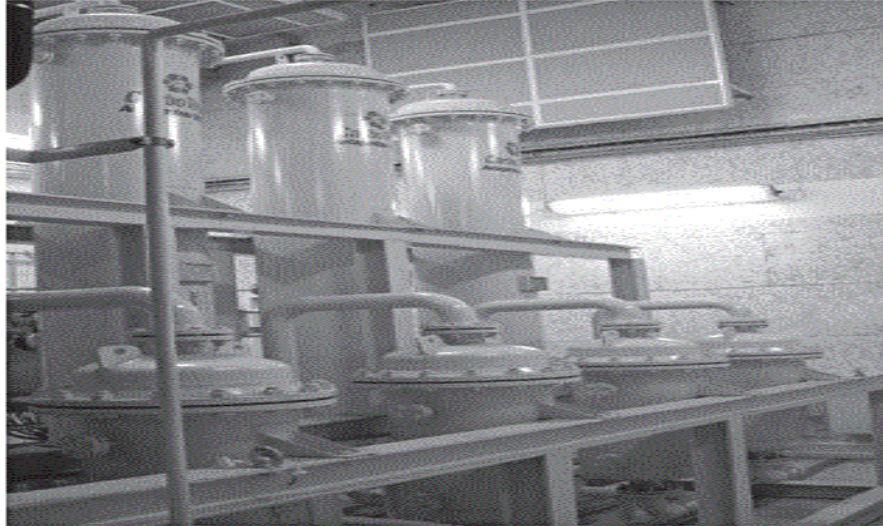
Figure 2.7. Installation for biomethane upgrading working in PSA technology, Helsingborg, Sweden
