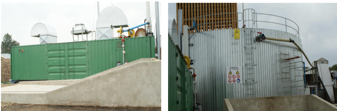
Figure 2.19: Jan Kempdorp abattoir- anaerobic digestion system
