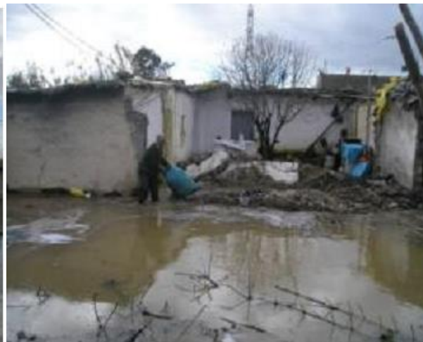
Photo 1: Partial destruction of a house in Douar Mchraa Kraym
