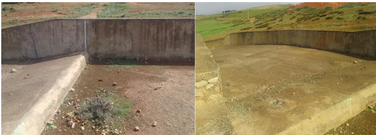
Photo 6: Oued Boufekrane dyke
