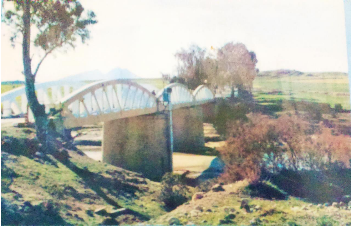
Figure 4. 1. Discharge station Mellegue k13 located on Mellegue river
