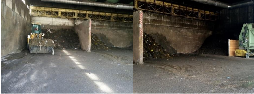
Figure 3. 1: Waste storage area
