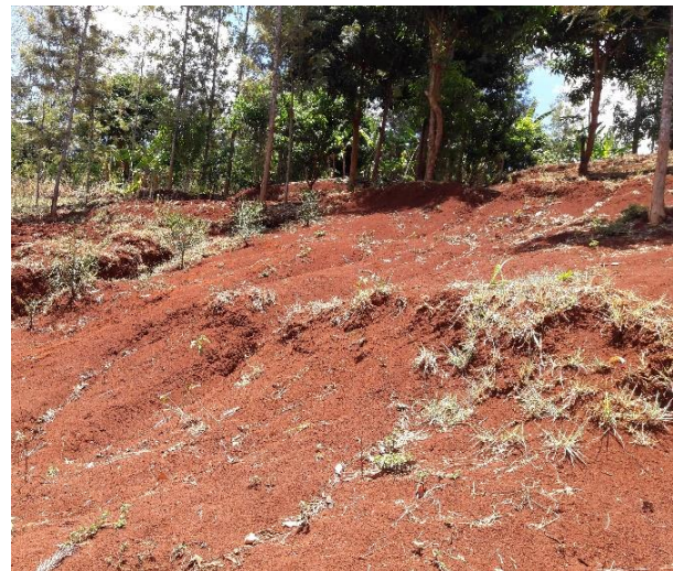
Figure 6. Collapsed terraces in Gatura village.
