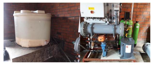
Preparation of Chlorine disinfectant by electrolysis of sodium chloride
