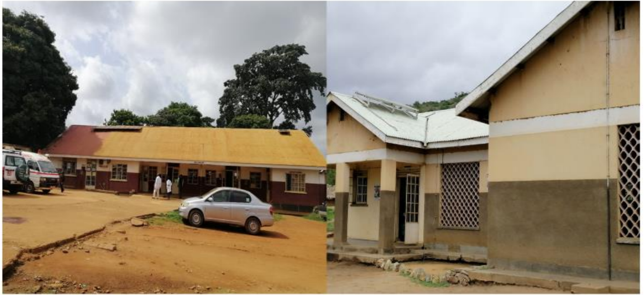
Photo Plate 5: A surgical annex ward at Hoima Main Hospital with solar back up and a rural health centre powered by solar PVs in Hoima District.
