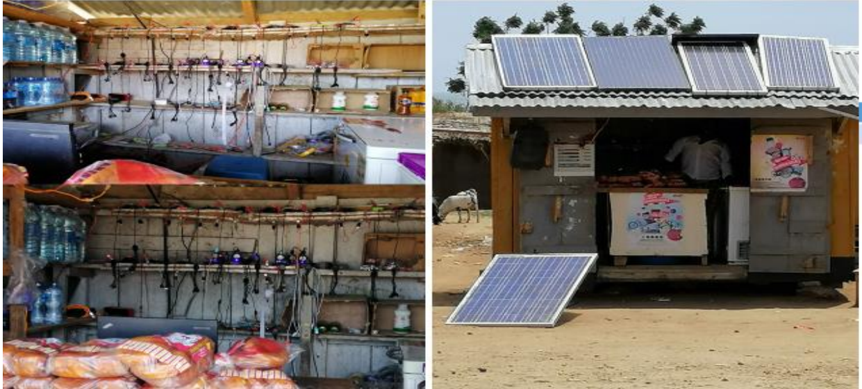
Photo Plate 3: A solar powered charging station with other commodities at Sebigoro village
