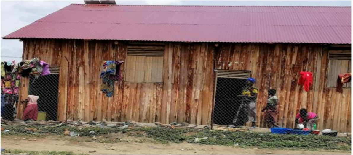
Photo Plate 7: A refuge reception centre powered by solar energy in one of the rural areas of Hoima District.
