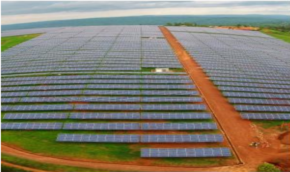
Figure 9. Gigawatt Solar power plant in Rwamagana district.
