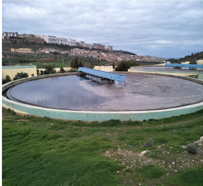
Figure 4.10: A clariflocculator
