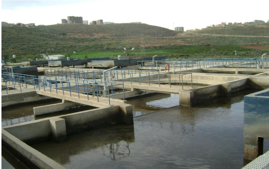
Figure 4.7: Nitrification and Denitrification Basins
