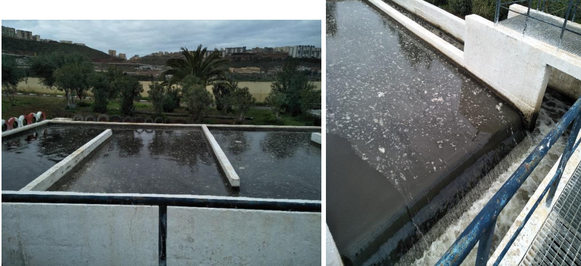
Figure 4.11: The disinfection basin
