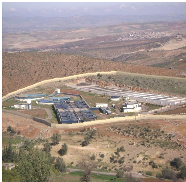
Figure 4.2: Panoramic image of the WWTP
