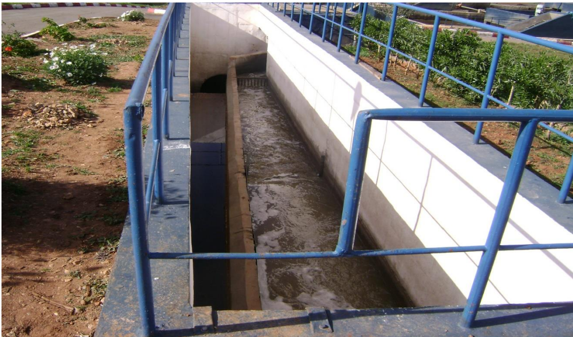
Figure 4.3: The storm weir
