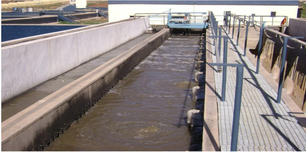
Figure 4.6: The sand, Grease and Oil removal units
