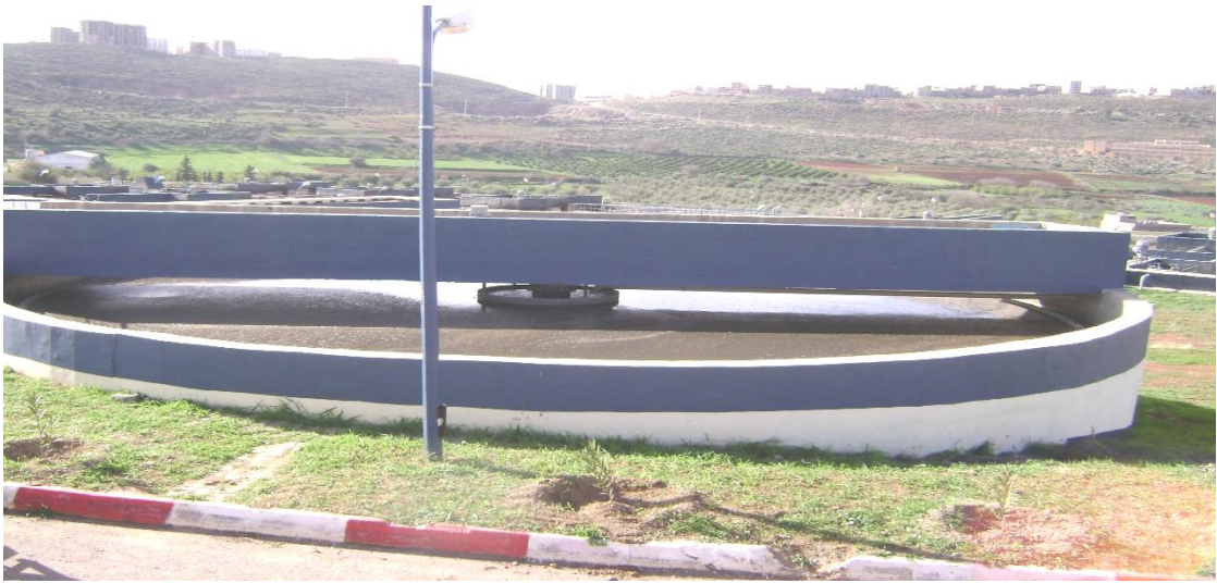
Figure 4.13: Sludge thickener
