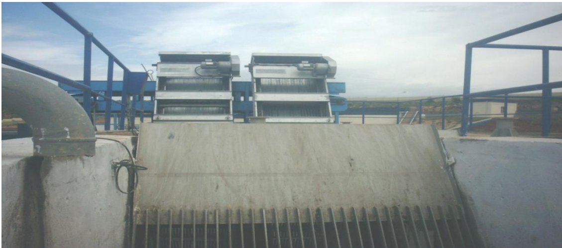
Figure 4.4: The Mobile Vertical Emergency Bar Screen
