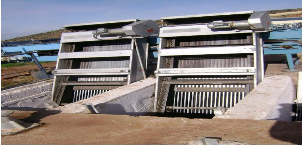
Figure 4.5: The coarse mechanical bar screen
