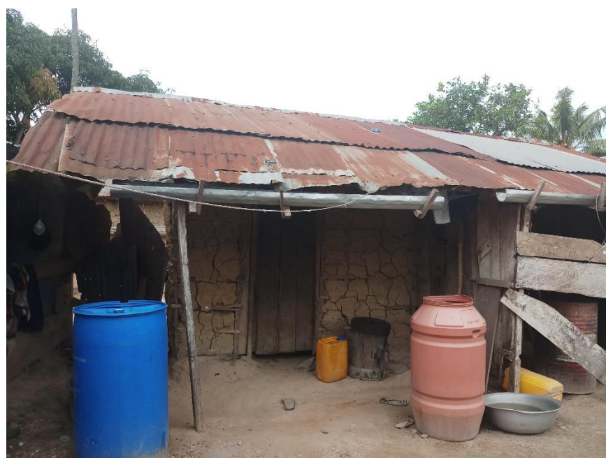
Figure 25: A typical rainwater harvesting system at Nyamebikyere (Field Survey, 2019)
