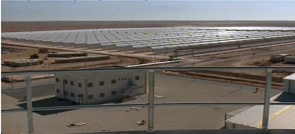
Figure 4-11: one of the world's first hybrid solar power plant is located at Hassi R'Mel
