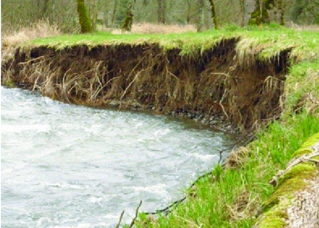
Figure 2.9: stream bank erosion
