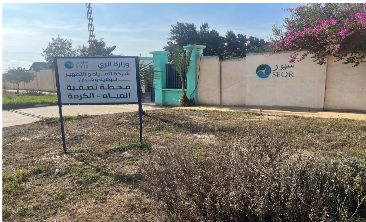
Figure 3.2: El kerma Wastewater treatment Plant
