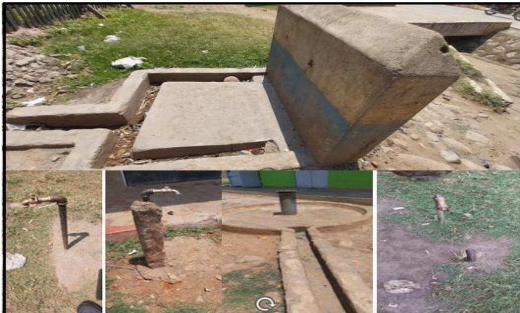
Plate 4.3.1.1: The broken (Malfunctioning) Water systems in different communities of Kasese Source: (Author’s Work, 2025)
