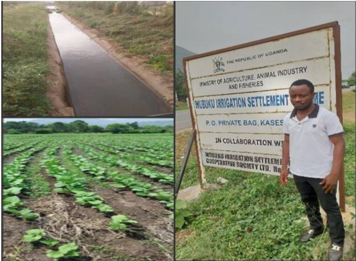
Plate 4.4.2: A field visit to the diverted River Nsebwe into the Mubuku irrigation Scheme Source: (Author's Work, 2025)
