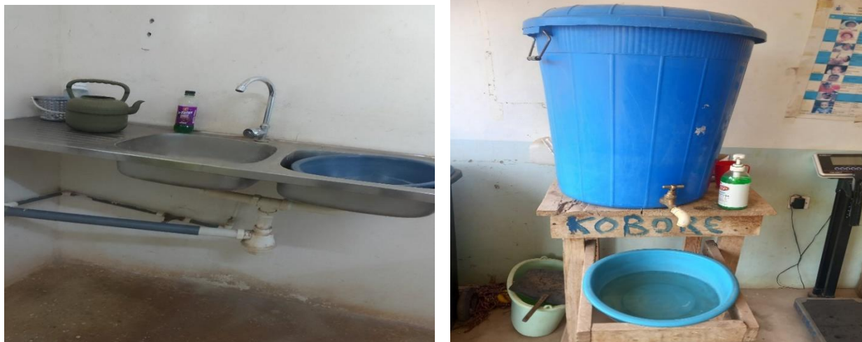
Figure 4: Pictures of Handwashing Facilities in some Health Facilities
