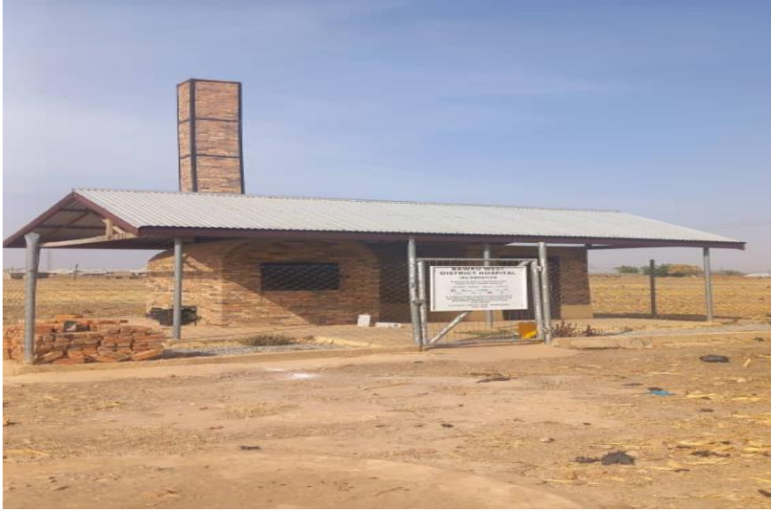
Figure 5: Picture of Bawku West District Hospital Incinerator
