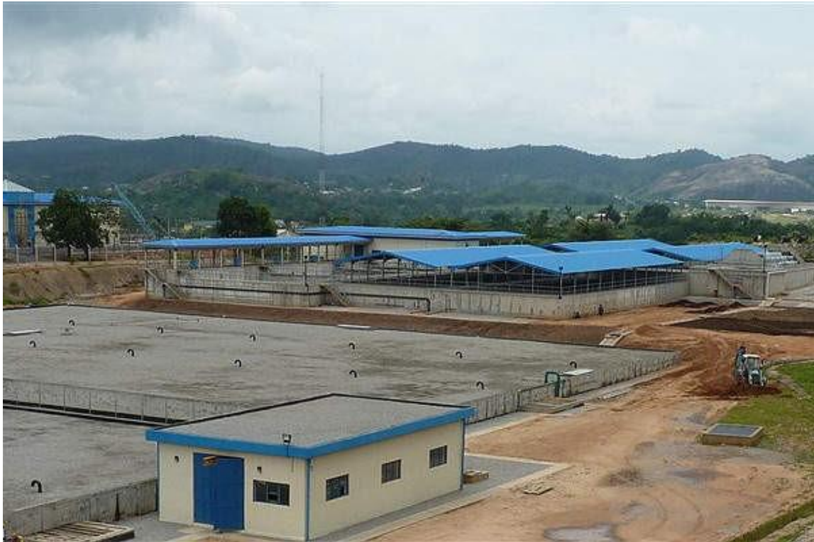
Figure 1.1: Lower usuman dam treatment plant, Abuja Image source: Biwater
