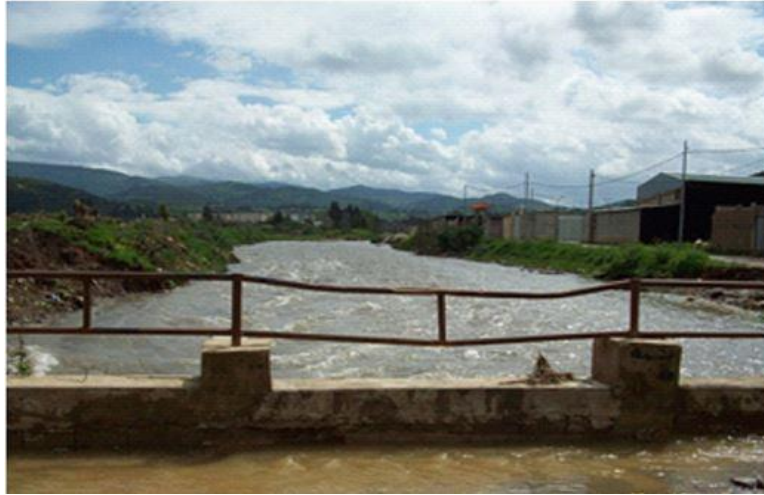
Figure 3: Bridge 2 (Br-2) during the flood event (Source: Otmane et al., 2024).
