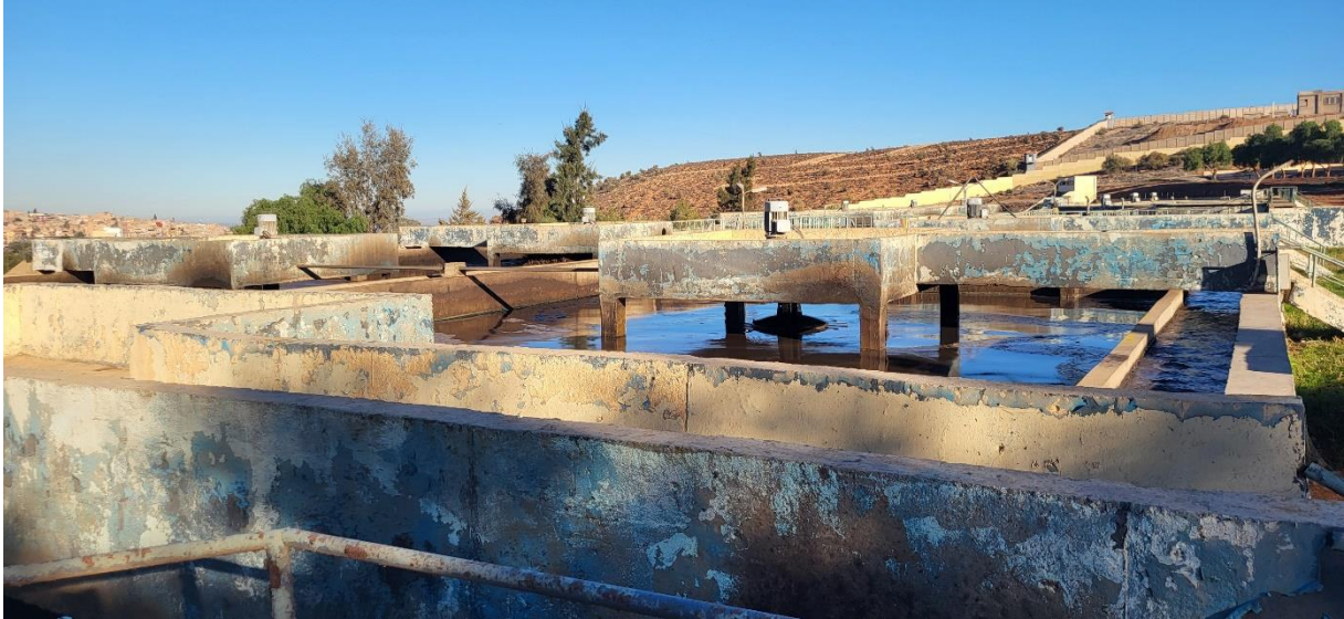
Figure 3. 7 Activated Sludge Basin
