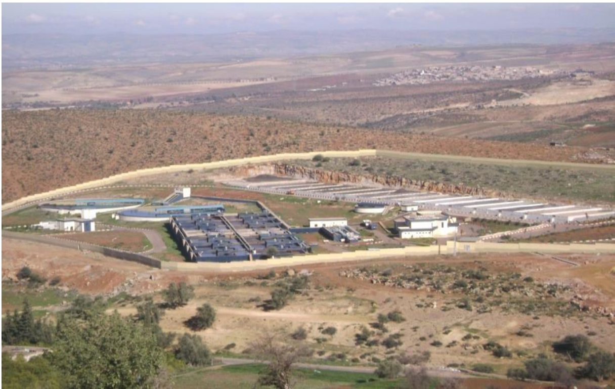
Figure 3. 2 Overview of Ain El Houtz WWTP
