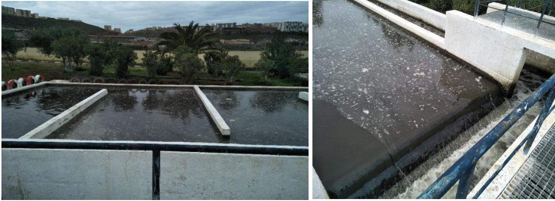
Figure 3. 10 Disinfection Basin
