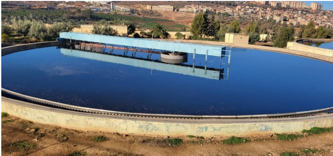
Figure 3. 9 Secondary Clarifier
