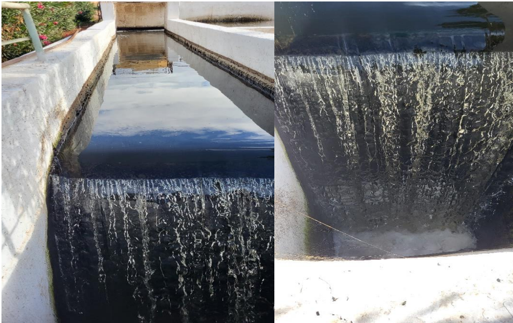
Figure 3. 11 Outlet from the WWTP
