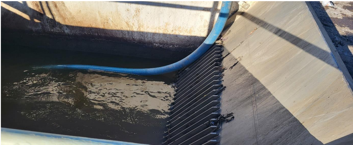
Figure 3. 4 Manual Coarse Screen
