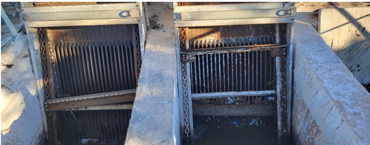
Figure 3. 4 Manual Coarse Screen
