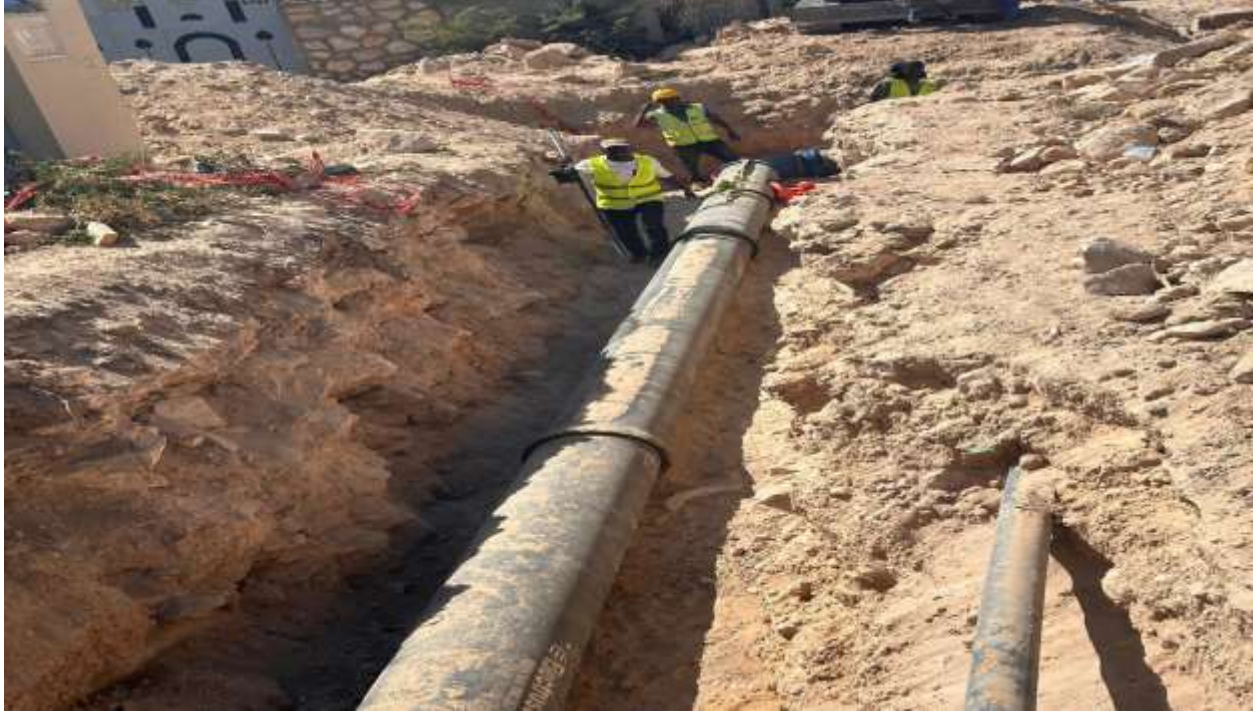
Photo 3. Hargeisa Urban Water Upgrade Project, (2024).
