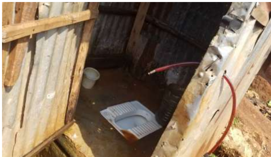
Figure 12: Squat pan toilet in Mvule zone in Namatata urban slum
