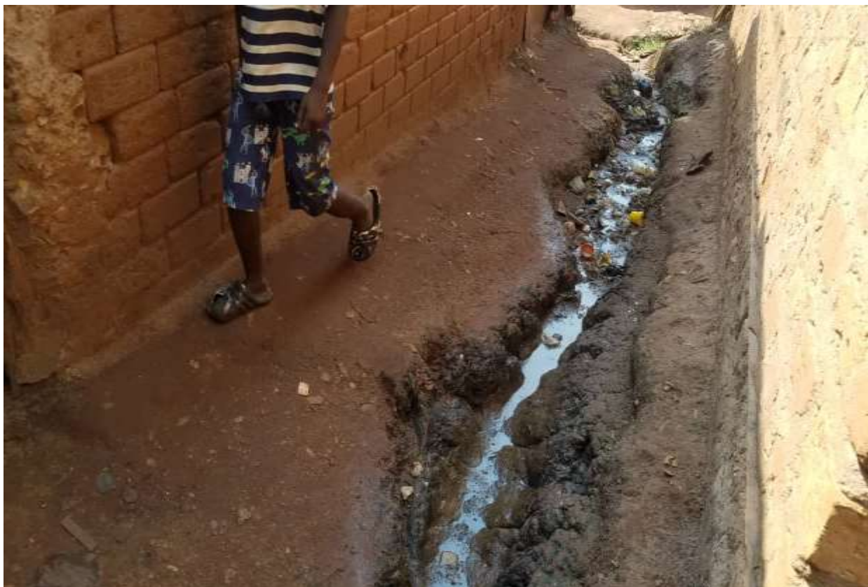
Figure 13: Waste water flowing in an open channel
