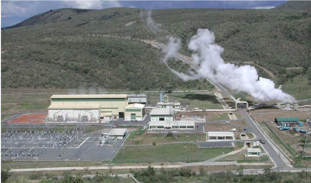
Figure 2.6- Olkaria II power station, commissioned in 2003
