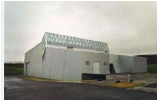
Figure 2.21 - Binary Kalina plant in Husavik, Iceland [29]
